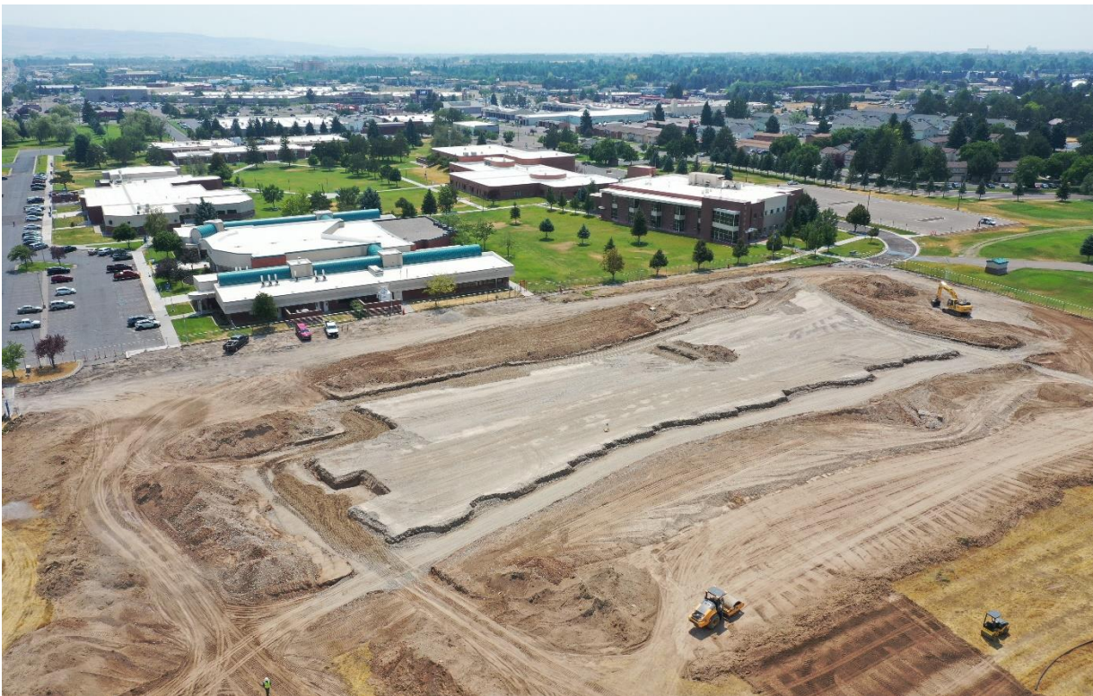
Future Tech Building groundwork has begun.
