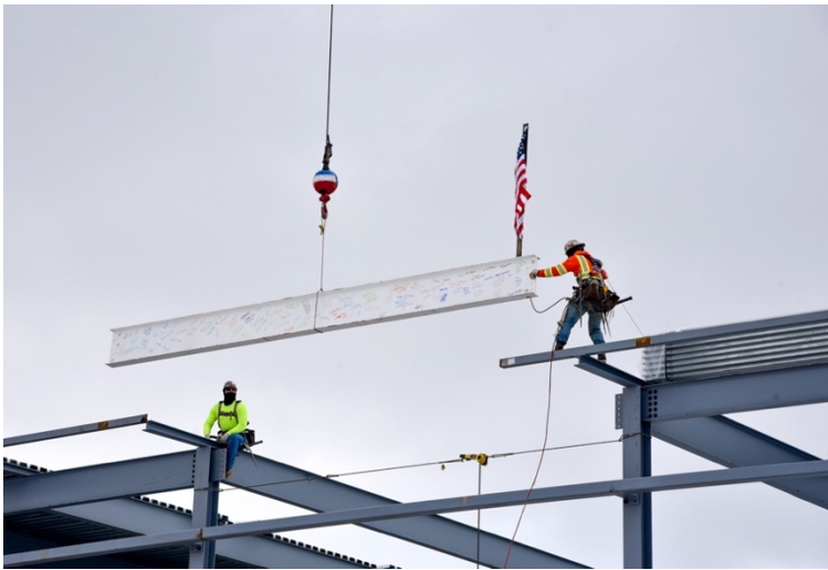
The final structural beam of Future Tech being installed.
